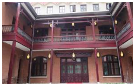
A century-old European style mansion was renovated at Taikoo Hui to maintain Shanghai's rich architectural history
