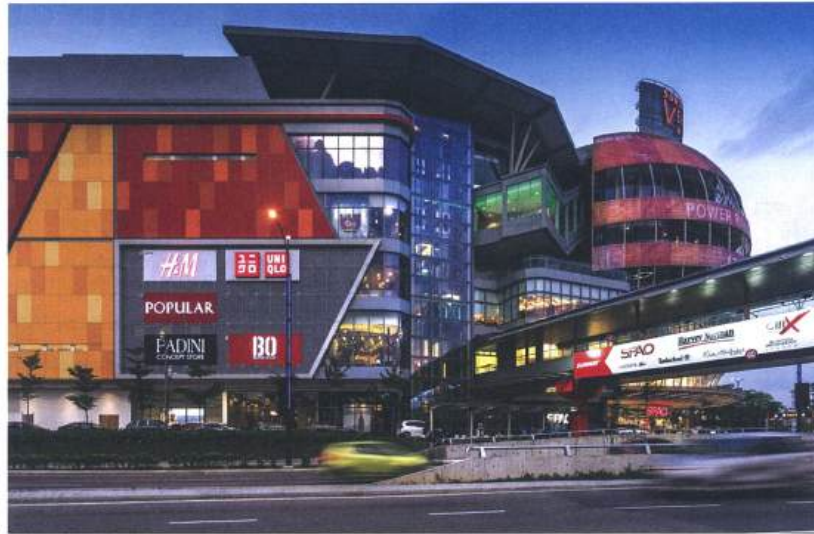
Sunway Velocity has an inviting and exciting frontage design that serves to draw shoppers
