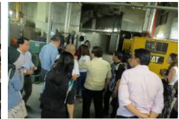
So, this is how a plant room looks like ...
