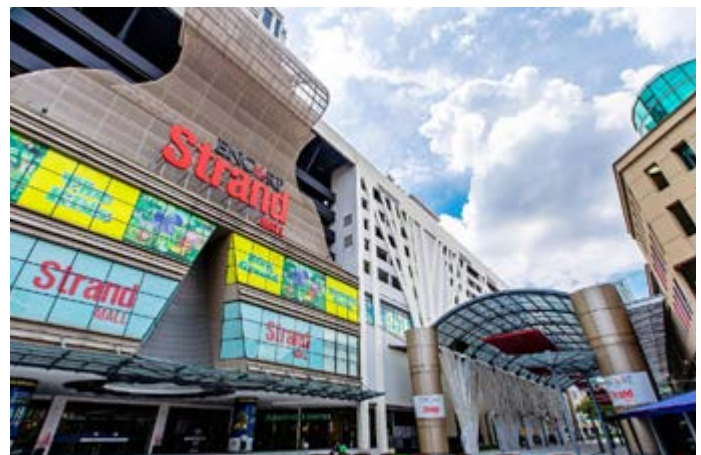
Rebranding and upgrading works ongoing at the mall
