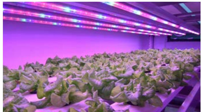
LED lights of red, green and blue designed for specific vegetable growth
