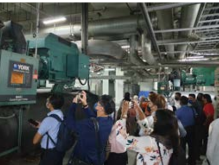
Participants of Operations module at the chiller room of Pavilion KL
